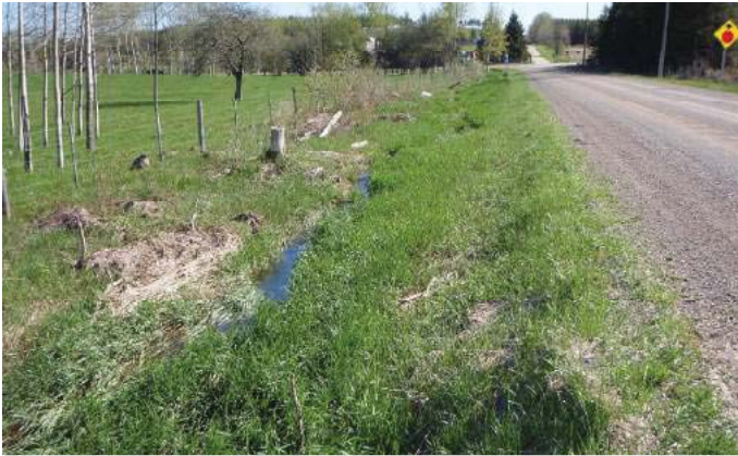
Meandering pattern forming within roadside ditch (Reach 12-169)
