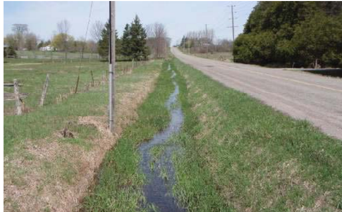
Meandering pattern forming within roadside ditch (Reach 15-104)
