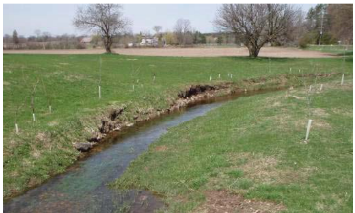
Minor bank erosion at downstream extent of straightened channel (Reach 15-093)
